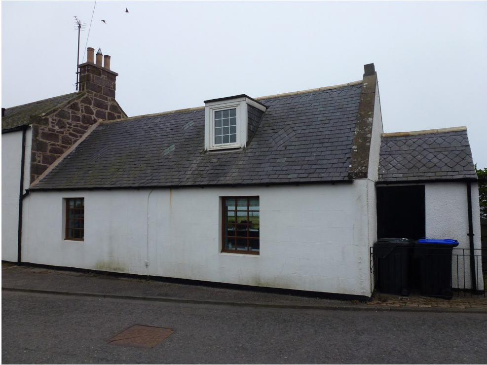
Pic. 2. School House, Cowie, Kincardineshire, Scotland. (Photograph by Jeremy Howard.)
