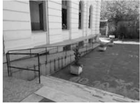
Pic. 5. Paula Soares State School access ramp (2016). From: author's private collection.
